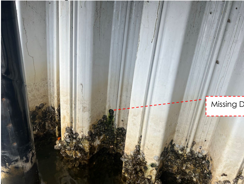
Photo #5 – Missing Drain.
