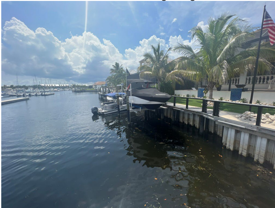
Photo #1- East End of Seawall. Beginning of Section 4.
