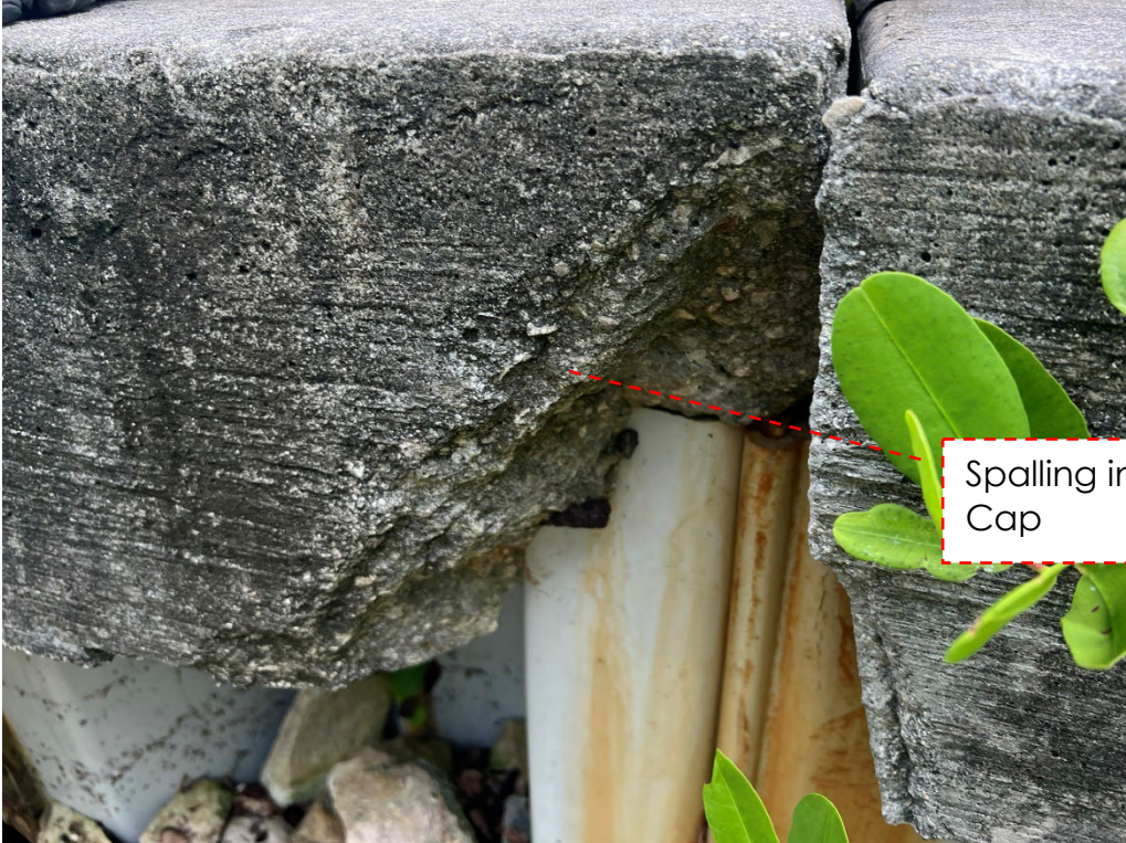
Photo #4 – Spalling in the Cap.
