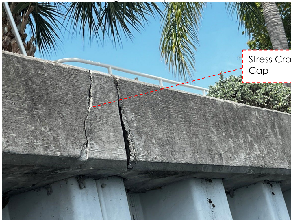
Photo #3 – Stress Cracking in the Cap.
