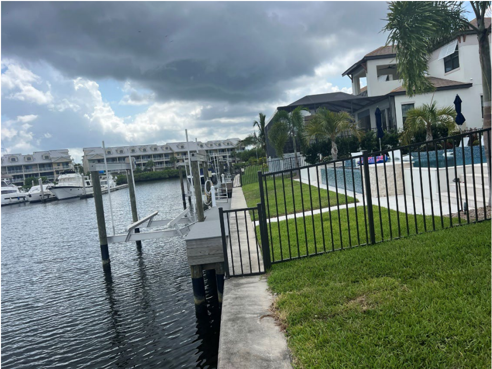
Photo #7 – Top View of the Wall Facing West.
