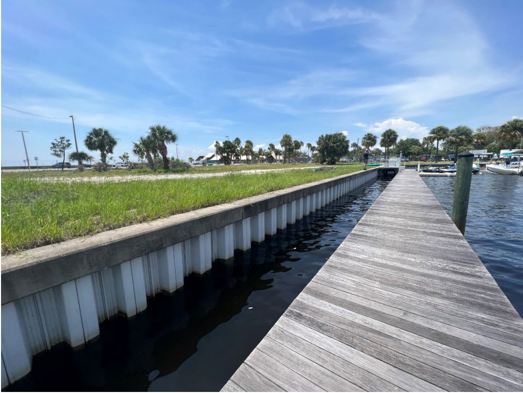
Photo #4 – Front View of the Seawall.
