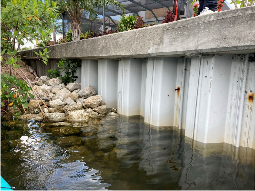
Photo #3 – Front View.
